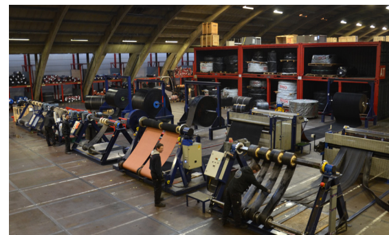
Conveyor Slitting & Winding Lines 5th line is fully installed and operational.
