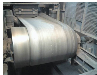
Before installation of Tru-Trac roller
