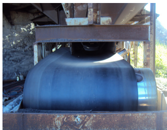
Before installation of Tru-Trac roller
