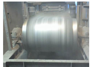
After installation of Tru-Trac roller
